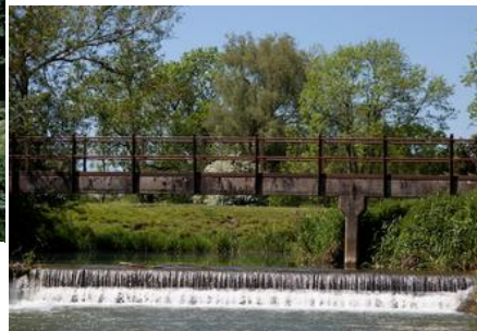
Weir, AMBER barrier Atlas
