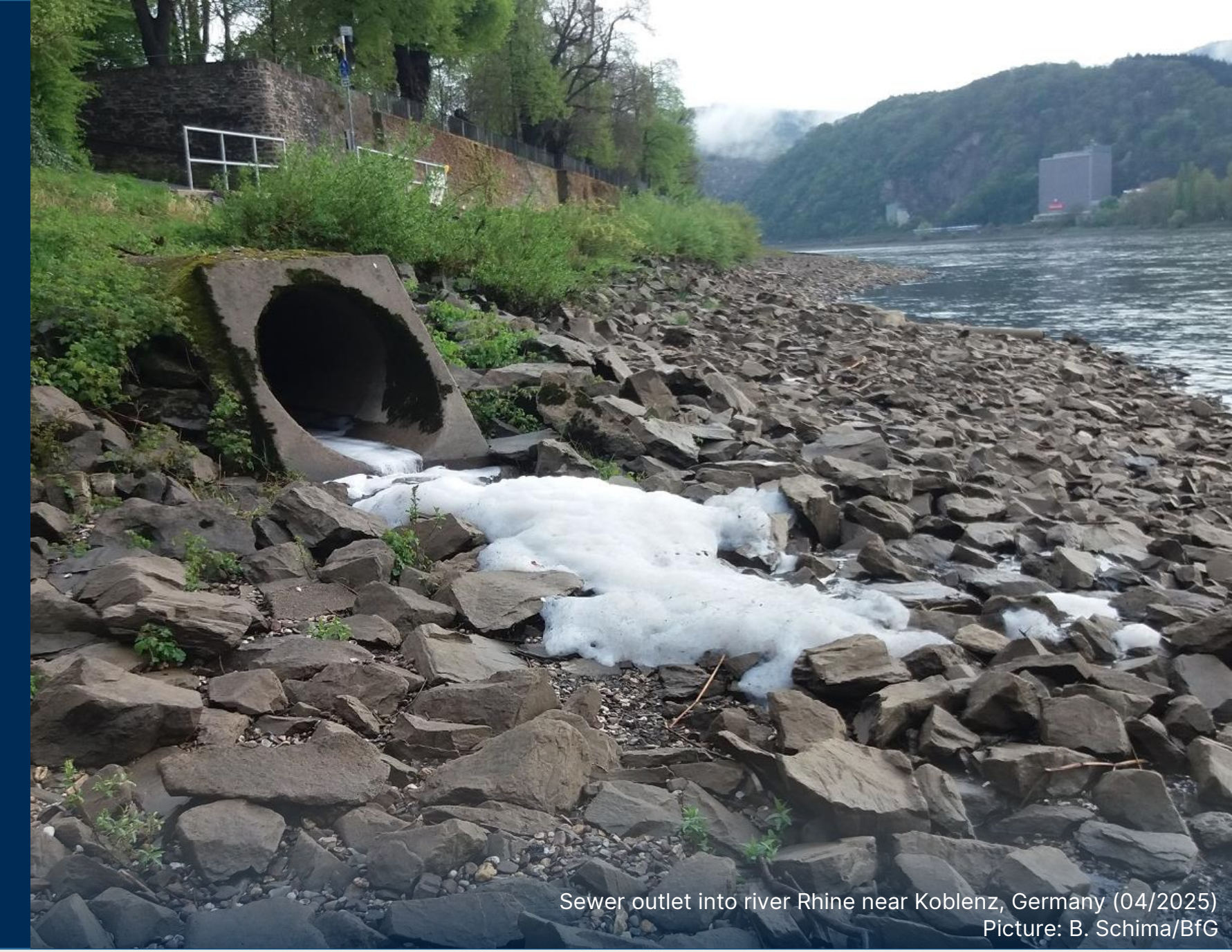
Sewer outlet into river Rhine near Koblenz, Germany (04/2025). Picture: B. Schima/BfG
