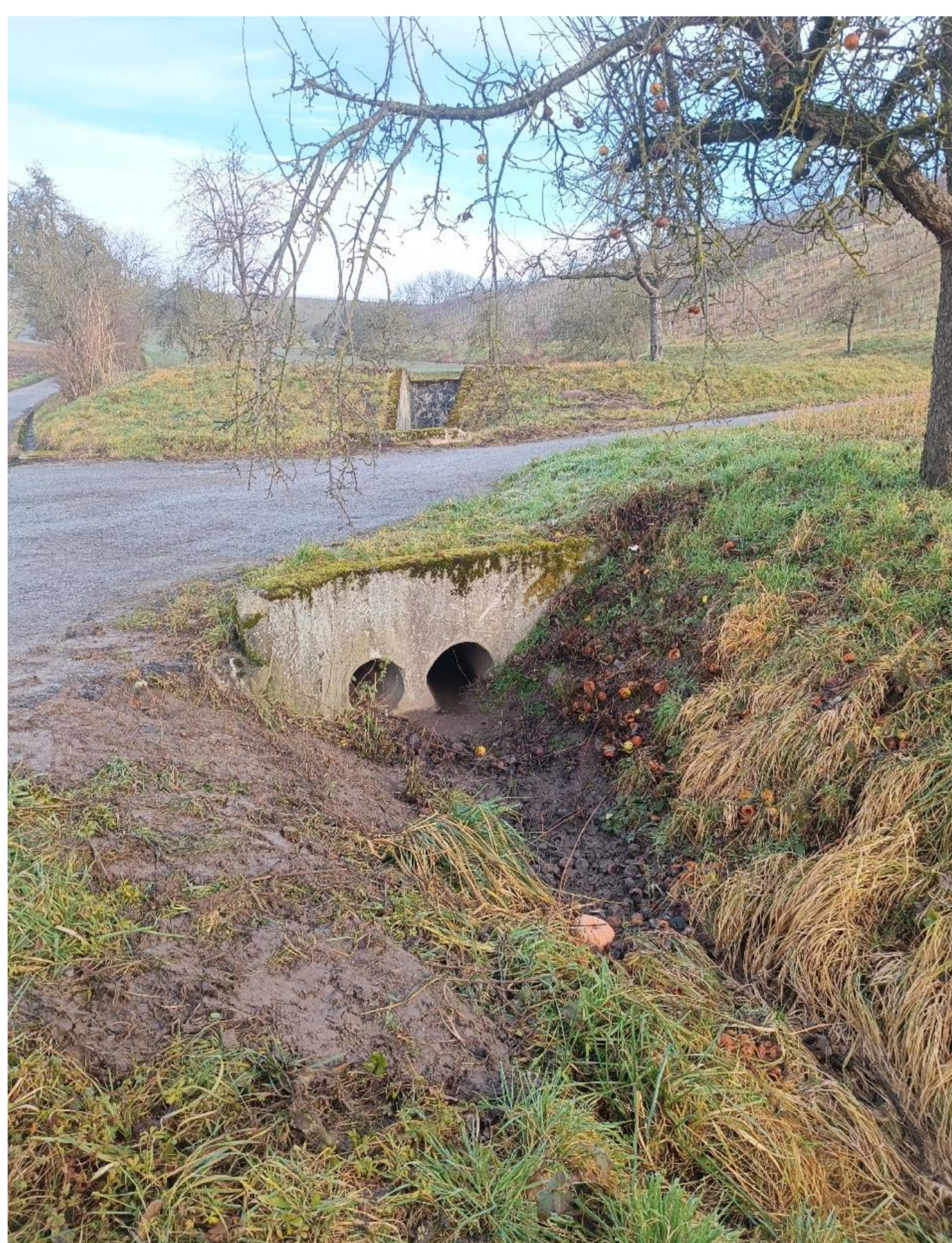
Fig. 1: Outlets from concrete channels and a large retention area drain into the Kohlbach via a ditch (A).
