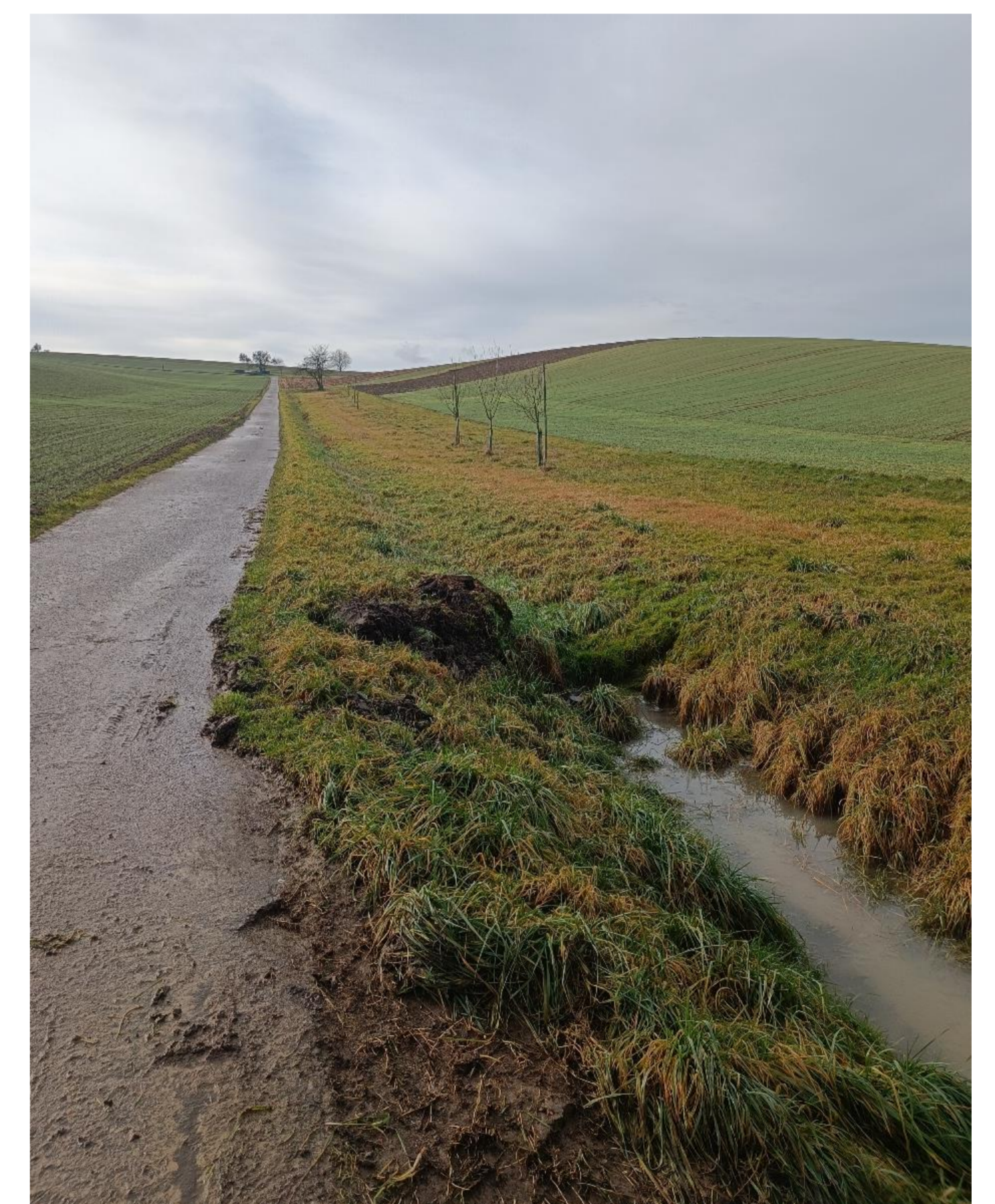
Fig. 3: Field ditch with turbid water and road with sediments (B).
